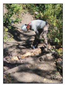
fixed tread issues and trail braiding, closed social trails, cleaned, and installed drainage structures, installed check steps, and inventoried campsites around the Lower Blue Lake.
