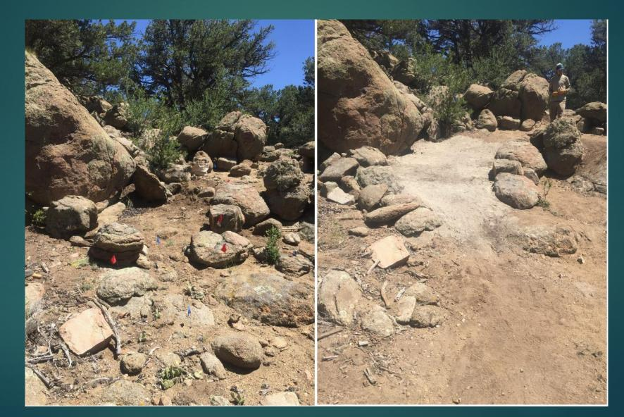
► Camp Elevation was a new trail construction project in 2019. The rock circled in red was moved to create more width and ended up being an important part of retaining the tread material.
