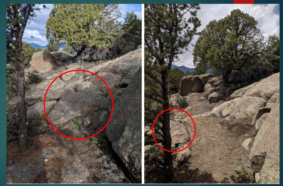
This picture shows the creation of a burmed turn for a mountain bike trail. All of the rocks seen in the before photo were used as the structure in the berm of the after photo.
