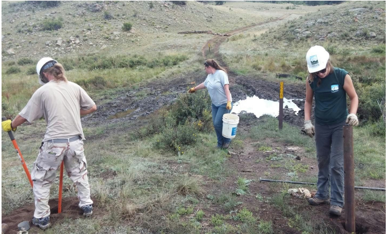
Above: Closing off an incredibly rutted out social trail in Badger Flats by spreading seed and digging holes for the fence posts. (Photo Credit: Michelle Holdener)
